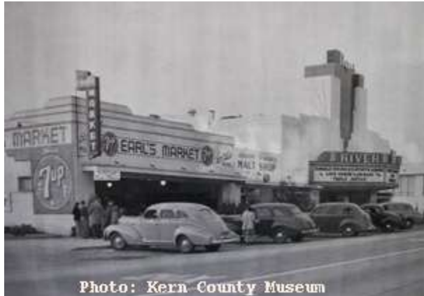
At right, River Theater on North Chester Avenue
