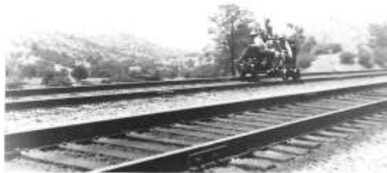
A section crew at the Loop, Dad's picture
